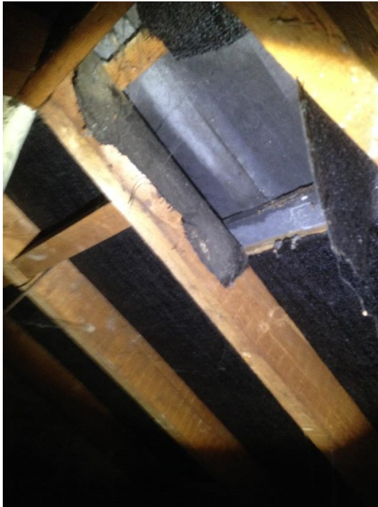
Figure 13: Torn roof felt lining exposing roof tiles, Void 1.
