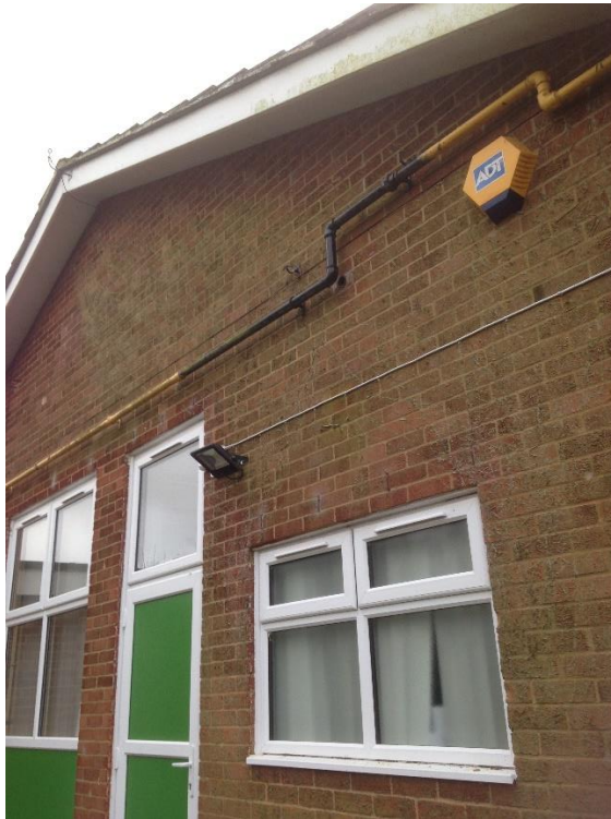
Figure 5: North western end of school building. Note hole in wall to left of security alarm box leading to loft void.
