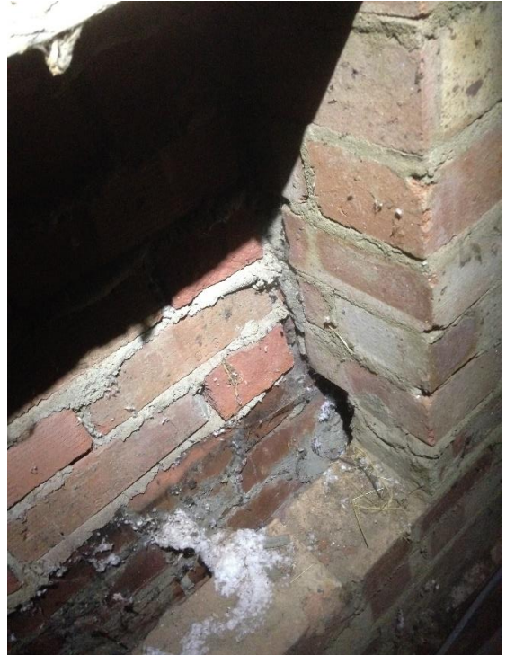
Figure 14: Evidence of cavity wall at north western gable, Void 1.
